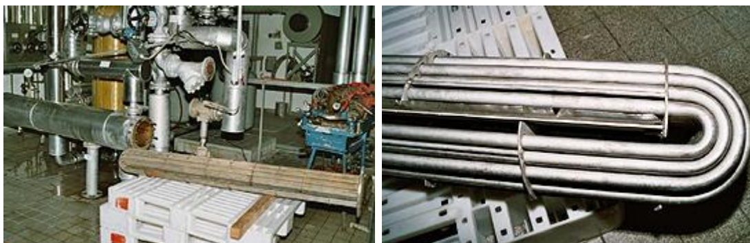
Hot water pipe (left)/ heat exchanger core and stainless steel guide to control internal flow (right)
