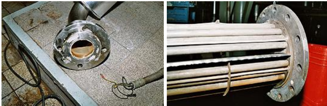
Hot water pipe (left)/ heat exchanger core and stainless steel guide to control internal flow (right)
